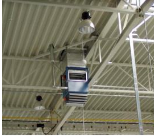
Fig. 5 Local ventilation (and heating) unit
